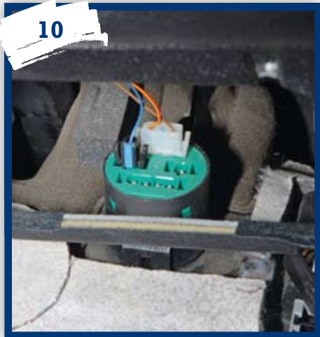
... while the wiring for the warning buzzer simply unplugs. Remember to disconnect the courtesy light for the footwell and you're done.
